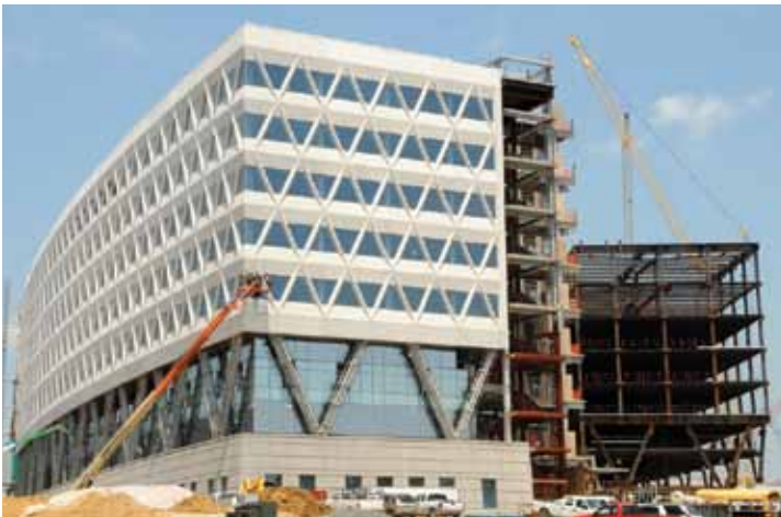
The new National Geospatial Agency campus being built on the former Engineer Proving Grounds at Fort Belvoir, Va., consists of two 1,100-foot-long, eight-story buildings connected by a six-story atrium. Built by the joint venture of Clarke/Balfour-Beatty, the project includes a large central utility plant, a parking structure, and a technical/data center.
