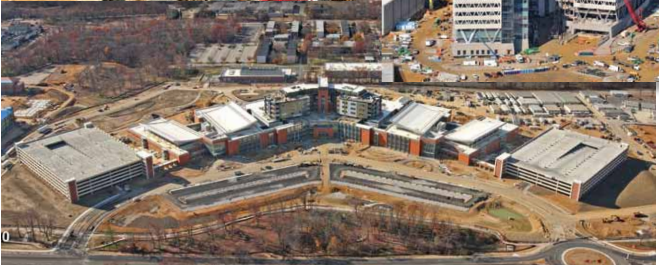
As a Base Realignment & Closure (BRAC) project, the National Geospatial Agency complex was on a fast track. To speed construction, precast concrete panels complete with wall assemblies were used to enclose the buildings. The design created distinctive architecture while meeting AT/FP requirements.
