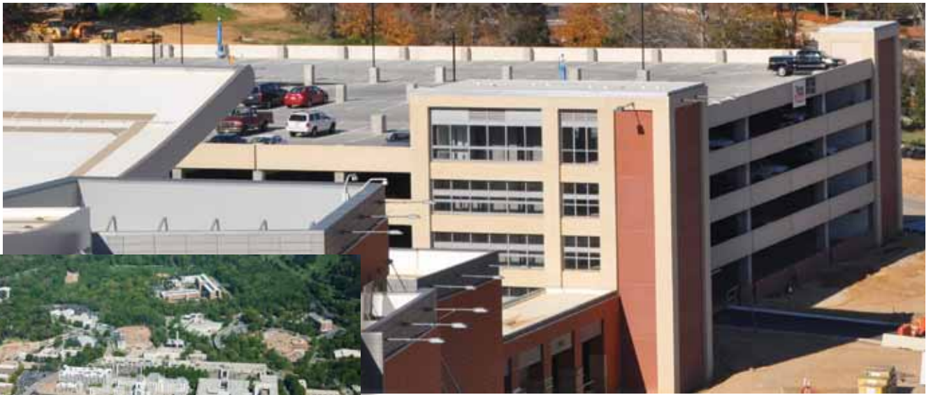
The new Fort Belvoir Community Hospital, a 1.3-million-square-foot facility, contains 120-inpatient beds and more than 650,000 square feet of out-patient clinical services. The campus also includes a six-story parking structure (left) and a five-story parking structure (right) with space for 3,000 cars.
